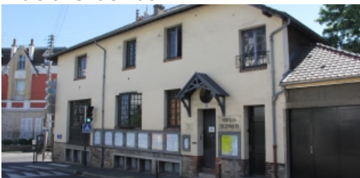
Direction des Services Techniques 1 avenue Rey de Foresta
